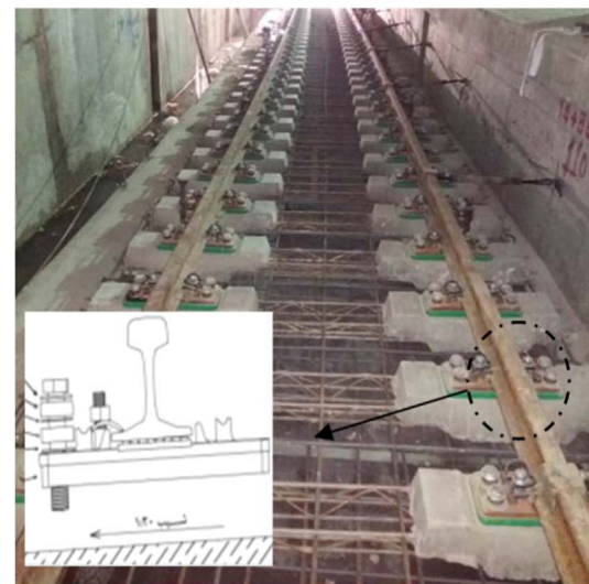
Fig. 16. Subway superstructure system (HRF) designed for Section 2 of Line 1 (Isfahan metro); currently under construction.
